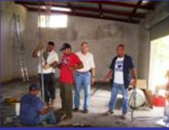
Installing the pump in the new bodega
