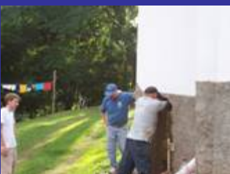
Working on the septic system at the farm
