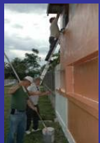
Painting the wall
