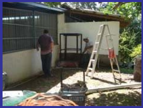
Construction of the new water tower
