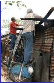
New roof at the Laurels
