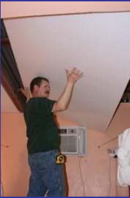
Inserting the Styrofoam in the clinic
