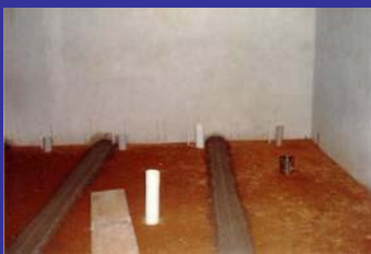
Inside new bathrooms
