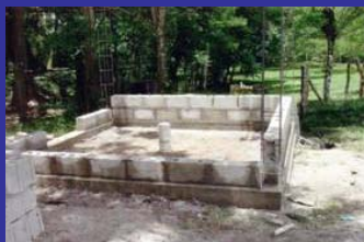
Beginning of the pump house
