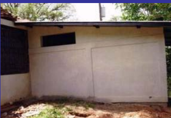
New men's showers and bathrooms next to the chapel
