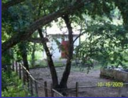
New well house on the farm
